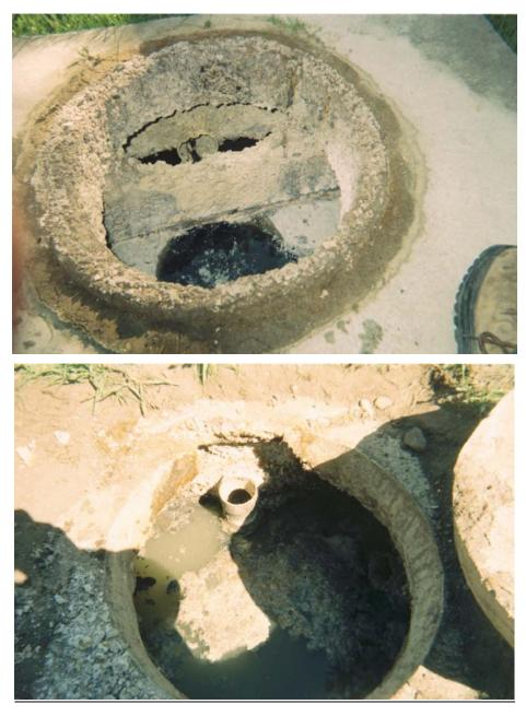
Figure 1. Corroded Outlet Baffles of two Tanks Receiving Water Softener Backwash – Does chloride accelerate the corrosion caused by H<sub>2</sub>S gas?
